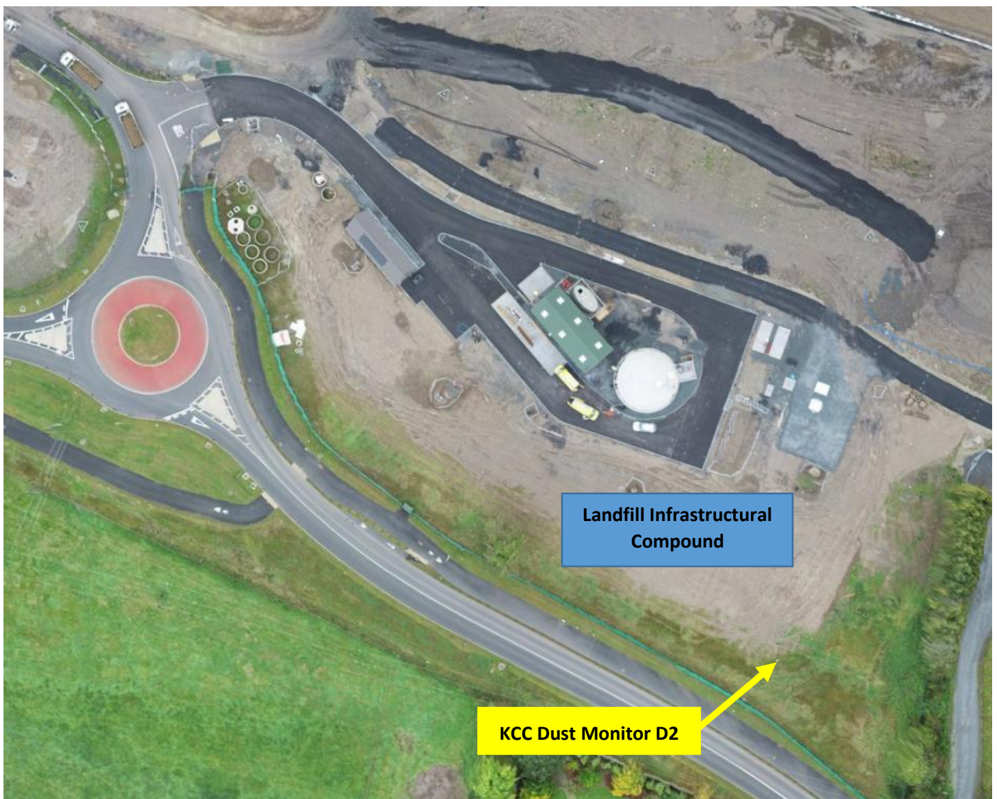
Figure 7-2 Landfill Infrastructural Compound
