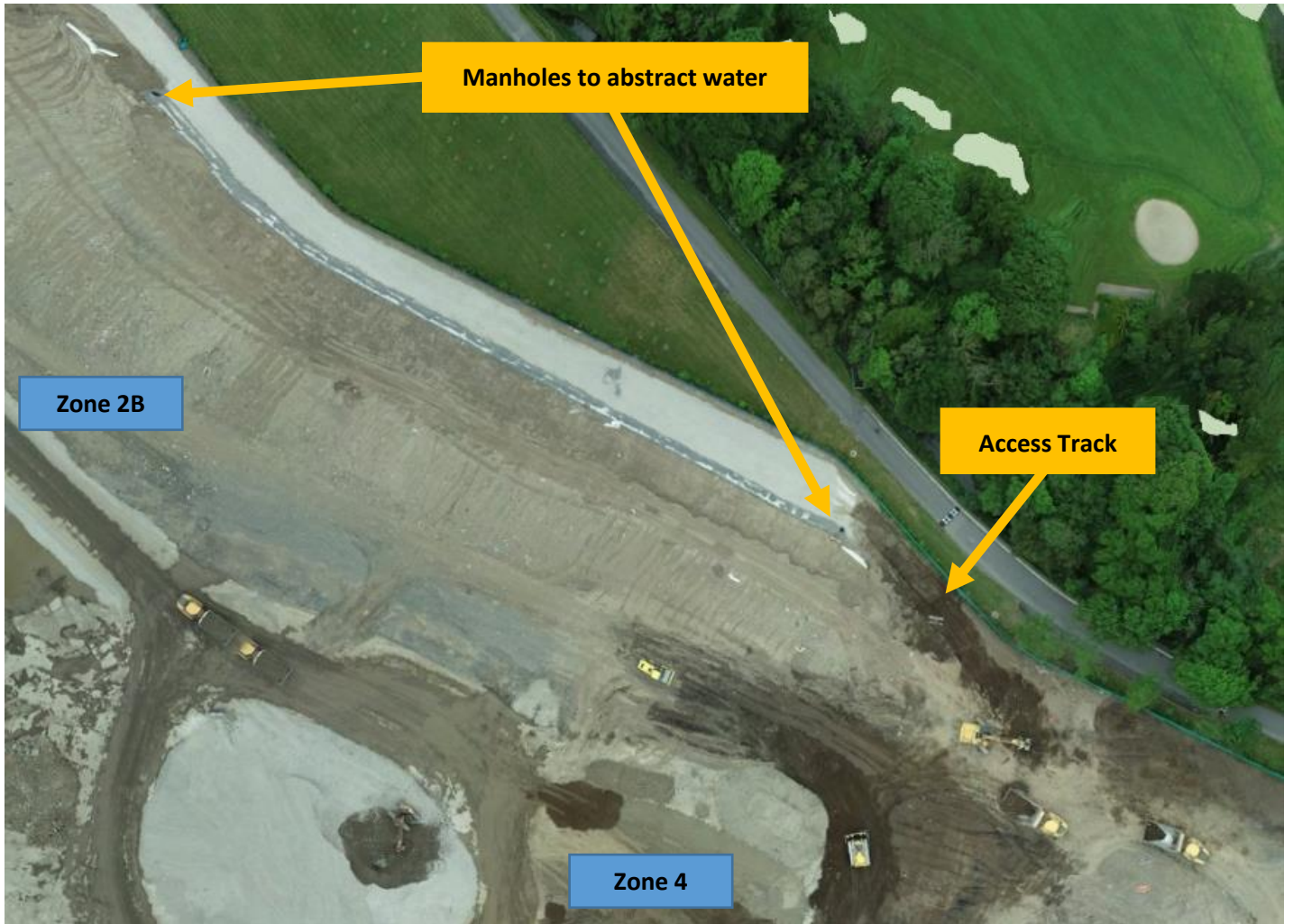
Figure 7-5 Groundwater - South Infiltration tunnel
