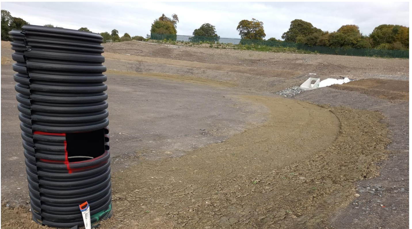
Figure 7-3 Standpipe installed at existing surface water lagoon location
